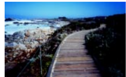
Figure 5. The boardwalk has raised edges to prevent users from accidentally leaving the path of travel.
