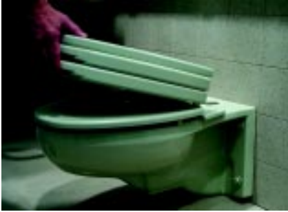
Figure 2. A toilet seat that is height-adjustable can be used by people of all sizes and ages.
