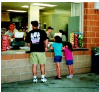
Figure 7. The height of the concession stand counter permits convenient use by customers of varying heights.
