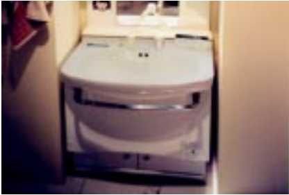
Figure 6. This lavatory has up and down controls that allow each user to adjust its height.
